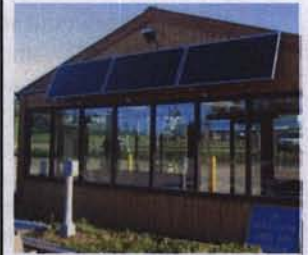
Solar panels on the Nenana parking lot bus shelter.
