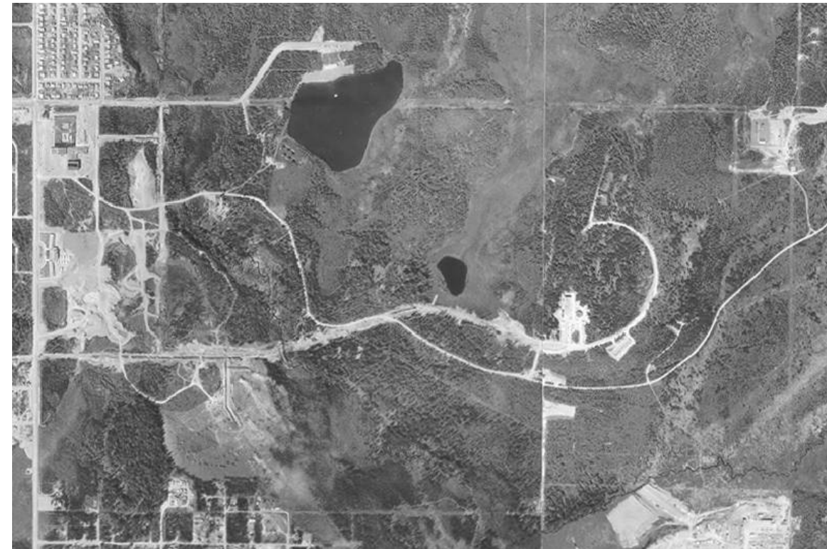
1960- Power lines were extended across Goose Lake.
