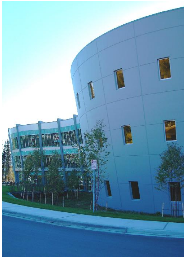
The new library addition is an imaginative example of northern sub-Arctic architecture.
