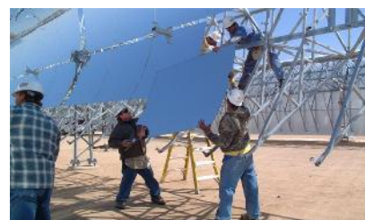
Figure 25.4. Andasol – a “100 MW” solar power station under construction in Spain. Excess thermal energy produced during the day will be stored in liquid salt tanks for up to seven hours, allowing a continuous and stable supply of electric power to the grid. The power station is predicted to produce 350 GWh per year (40 MW). The parabolic troughs occupy 400 hectares, so the power per unit land area will be 10 \text{ W/m}^2 . Upper photo: ABB. Lower photo: IEA SolarPACES.
