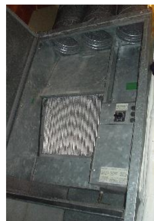
Figure E.11. The Heatkeeper's heat-exchanger.
