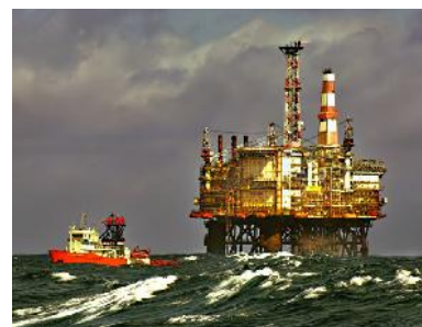
Figure 10.4. The Magnus platform in the northern UK sector of the North Sea contains 71 000 tons of steel. In the year 2000 this platform delivered 3.8 million tons of oil and gas – a power of 5 GW. The platform cost £1.1 billion. Photos by Terry Cavnar.
