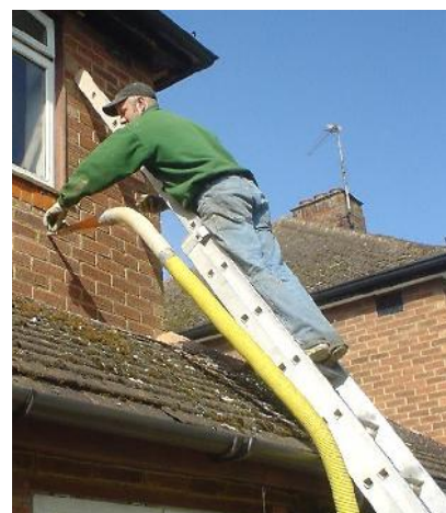
Figure 21.5. Cavity-wall insulation going in.
