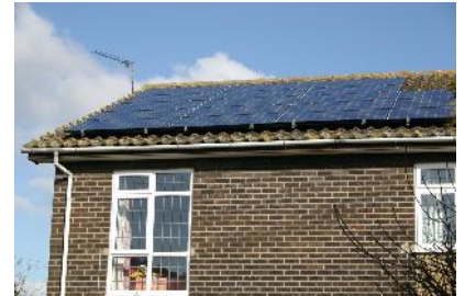
Figure 6.5. Solar photovoltaics: data from a 25\text{-m}^2 array in Cambridgeshire in 2006. The peak power delivered by this array is about 4 kW. The average, year-round, is 12 kWh per day. That's 20 W per square metre of panel.
