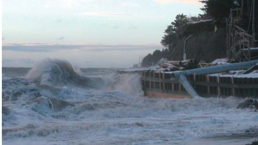
The Homer seawall was battered by waves during a winter storm when the wall was still under construction. (Photo by Carl Schoch)
