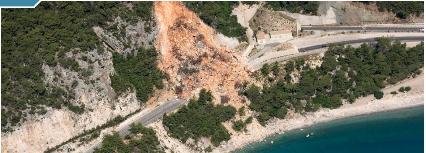
Landslide blocking a road in California
