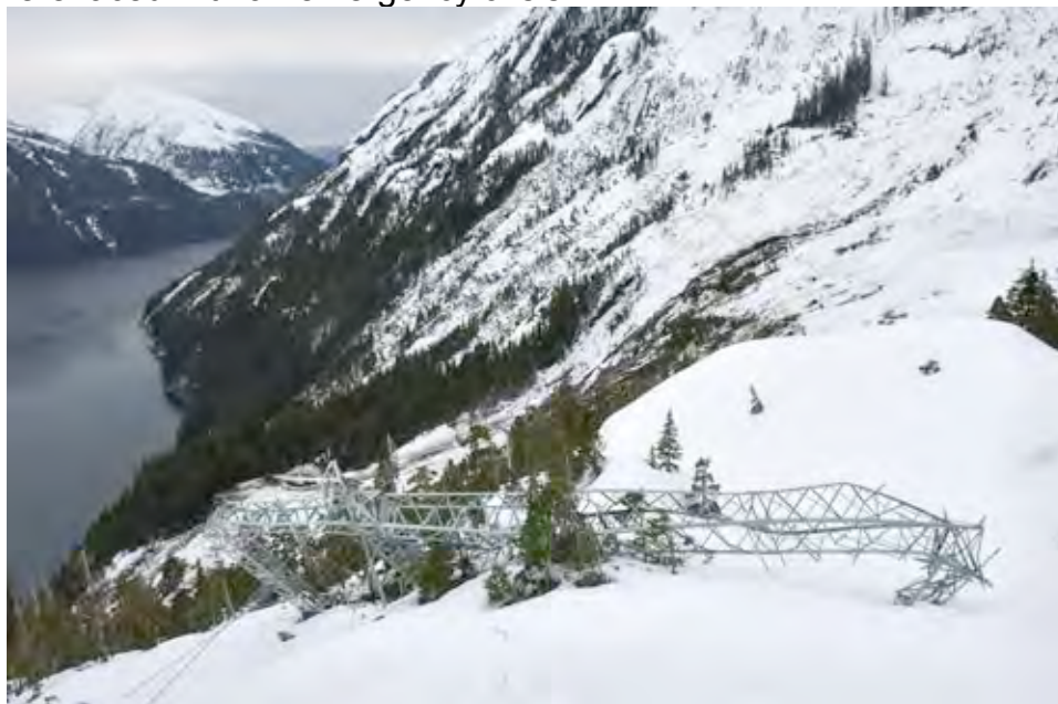
Figure 4. Transmission Tower Knocked Down by Spring Avalanche. 94
